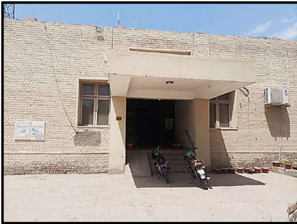
“Inside view of the property”
